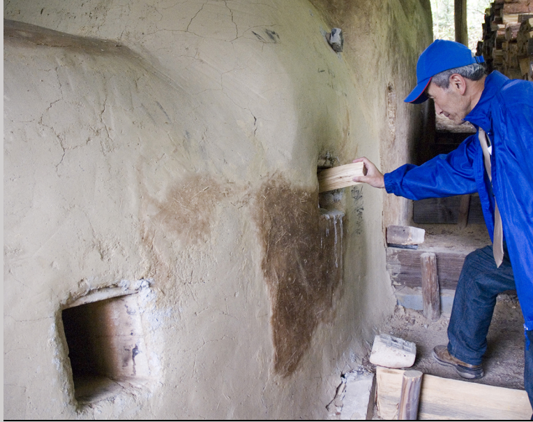
Figure 6.16d How wood would be stoked into a chamber of the noborigama kiln at the Shigaraki Ceramic Cultural Park, Japan (photograph by Carol Ventura, 2006).
